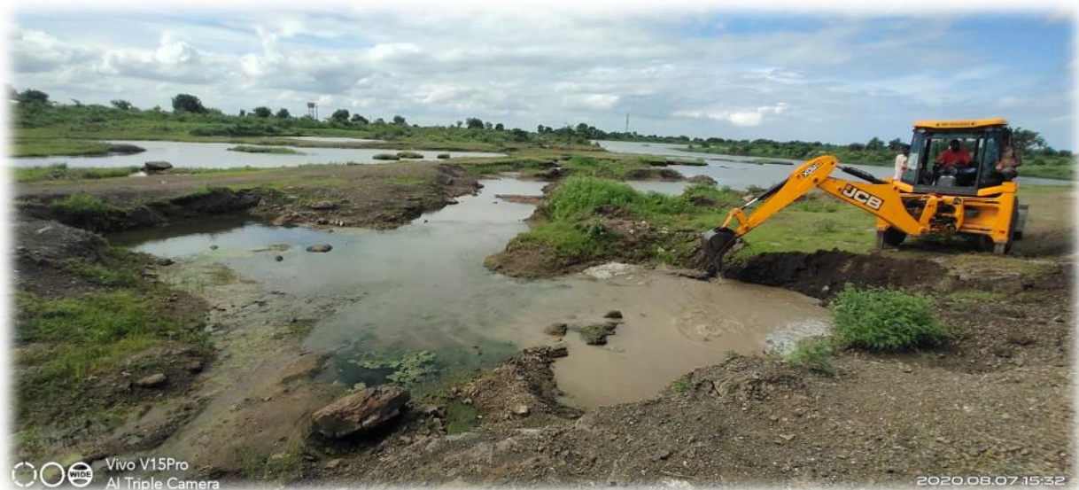
Picture 6: Stream desilting work in Lonje village
