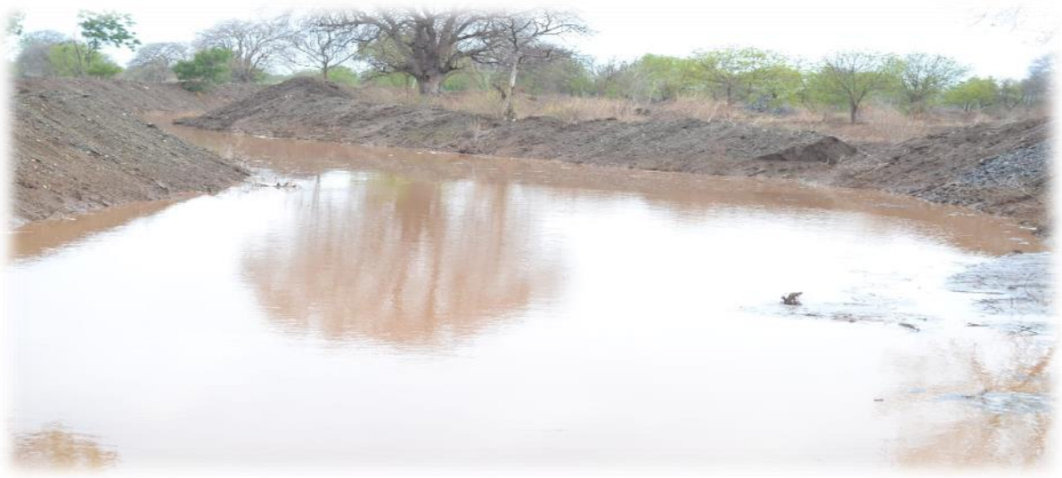
Picture 2: Rainwater in stream after desilting, widening and deepening activities
